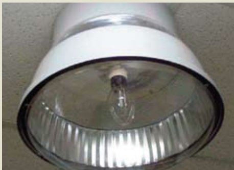
Figure 6. A KIM PGL luminaire can be used for lighting in precast and post-tensioned concrete parking structures.
