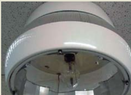
Figure 5. A Lithonia PGR luminaire can be used for lighting in precast and post-tensioned concrete parking structures.
