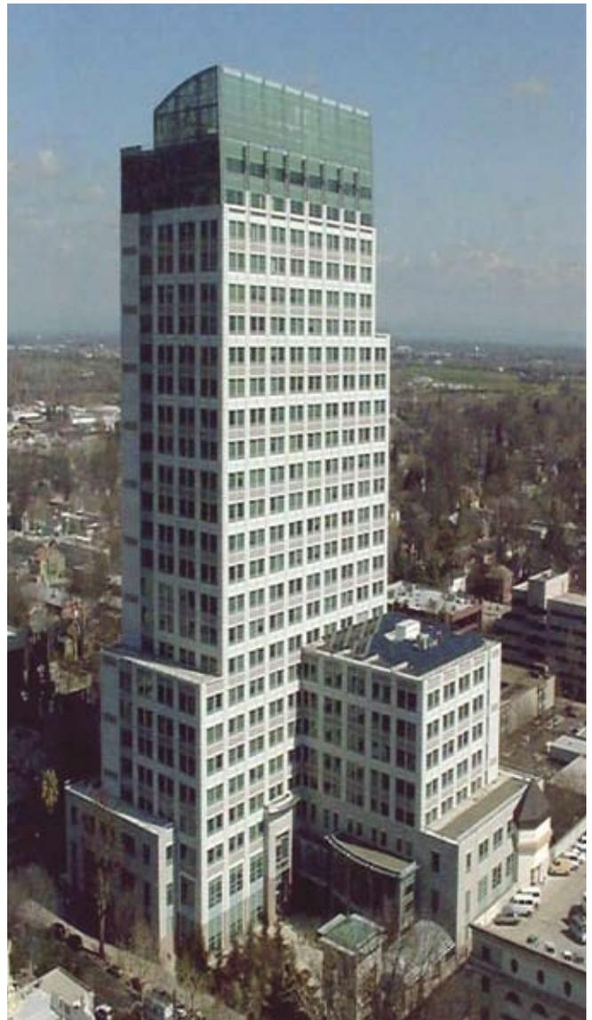
**Fig. 2.** The Joe Serna Jr. California EPA Headquarters—a 27-story LEED Platinum-certified office building in downtown Sacramento—has precast concrete panels with punched openings. The panels were pre-mounted, glazed, and caulked at the precast plant after casting.
