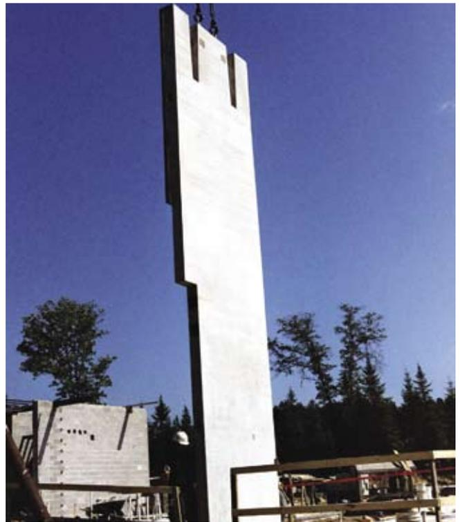
**Fig. 5.** Precast concrete panels provide effective sound barriers separating buildings from highways or industrial areas from residential areas.
